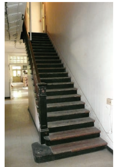
The open stair in the Main Building.
