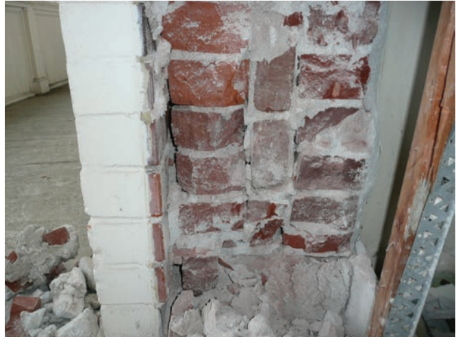
Exterior brick wall internal construction.
