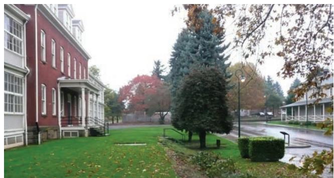
The east yard, looking north.
