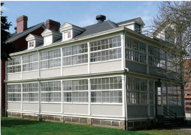
Northeast corner of the North Wing.
