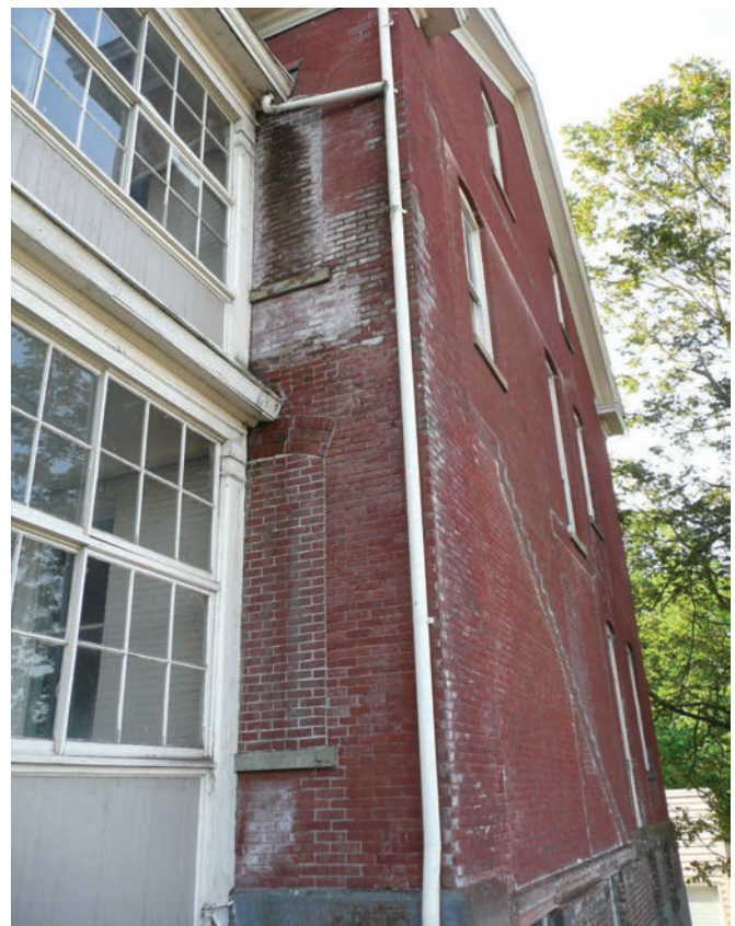
Northwest corner of the Annex.
