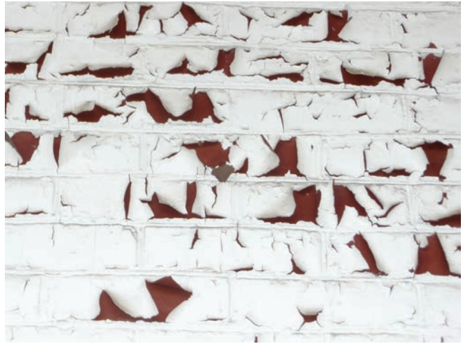
South Wing wall, with white paint applied over red mortar wash.
