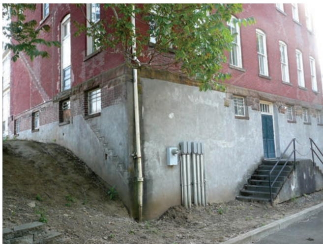
Southwest corner of the Annex.
