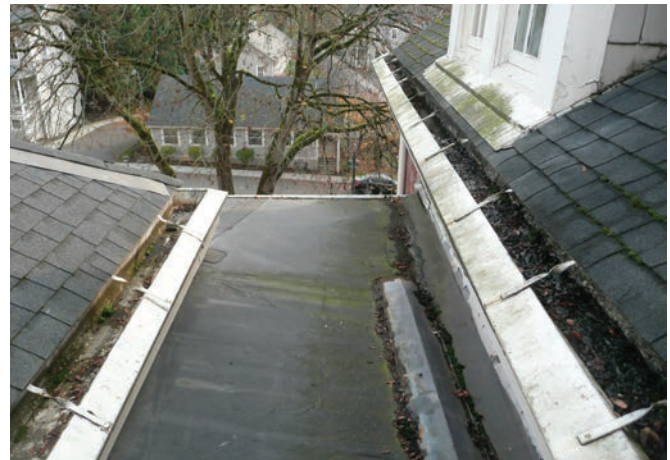
Built-in gutter system of the South Wing and the Annex.
