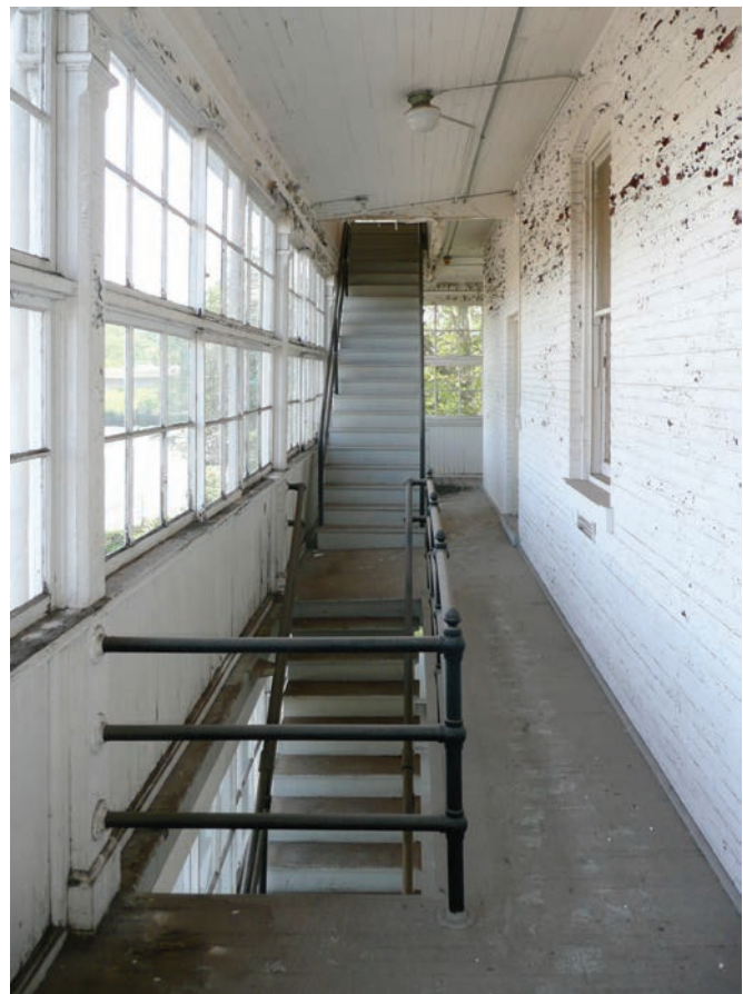
Porch stairway at second floor of the North Wing.
