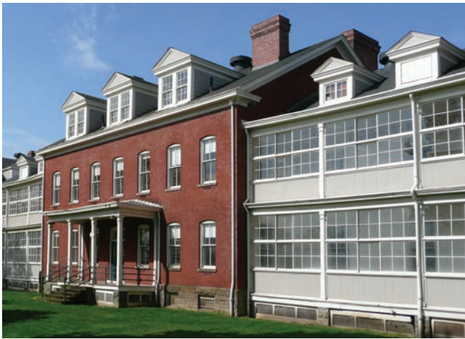
The east roofline.
