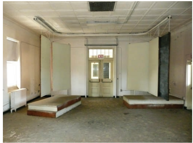
Second floor room in South Wing.
