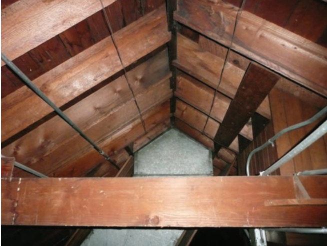
Roof framing at attic.
