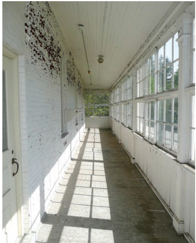
Interior condition of the North Wing porch.
